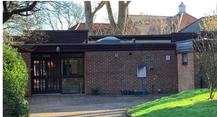
The existing church hall
