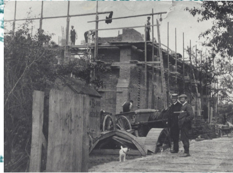
St John's under construction. © Harpenden and District Local History Society.
