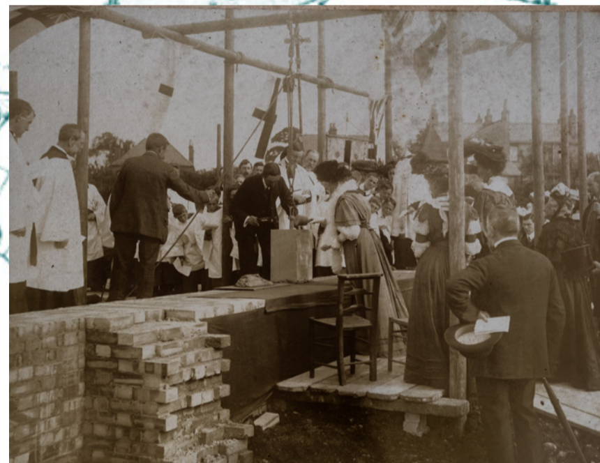
St John's foundation stone laid 27th July 1907.
